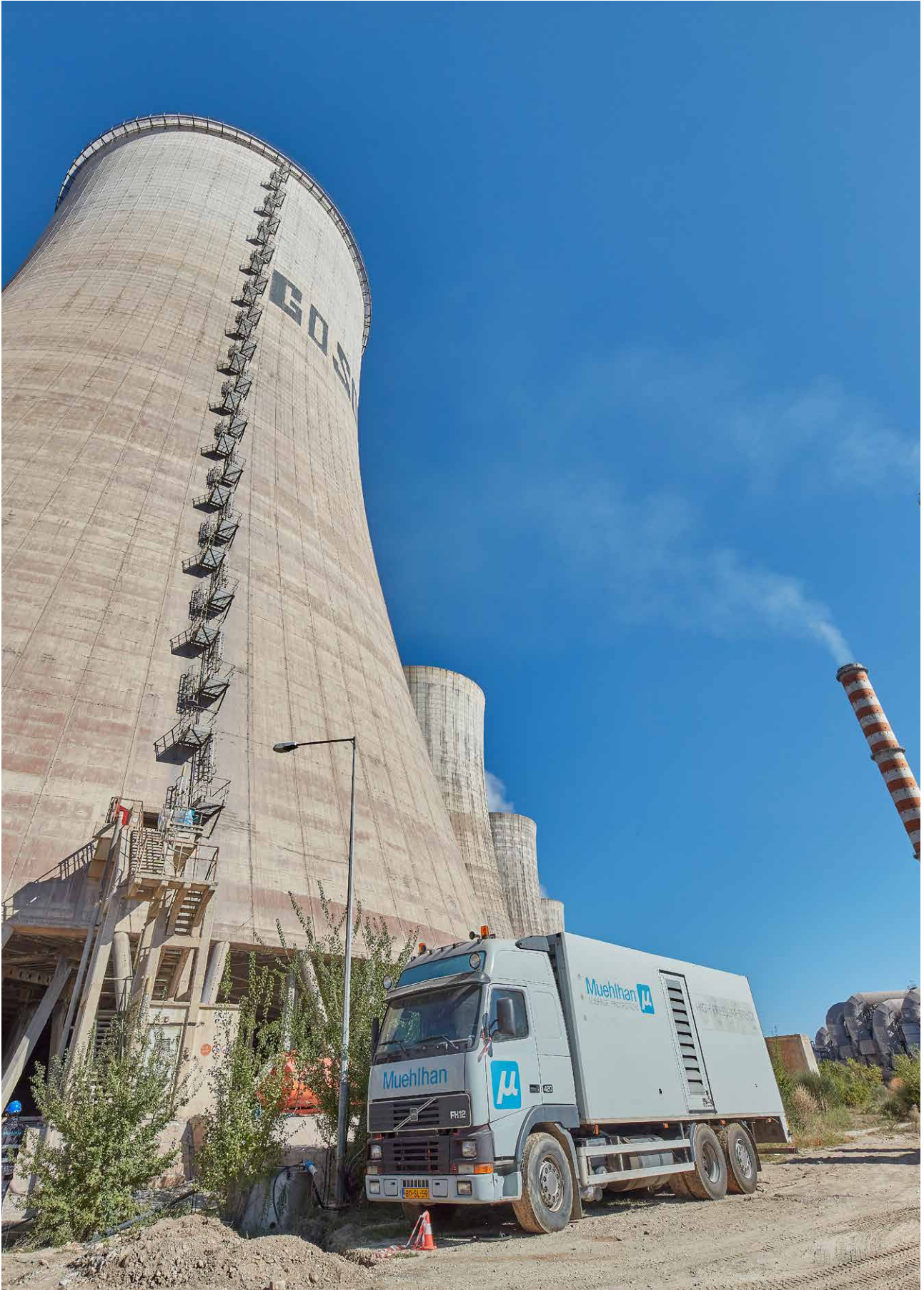
Work on a cooling tower in Greece
