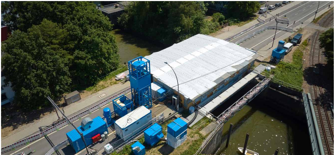
Maintenance work on a bridge
