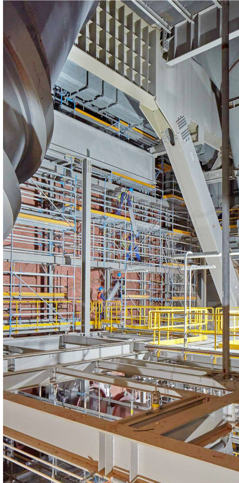
Scaffolding work on an industrial plant in Greece
