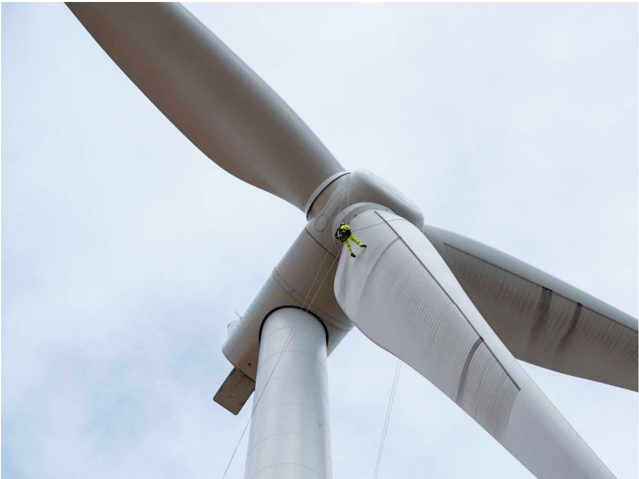
Inspection of rotor blades on a wind turbine
