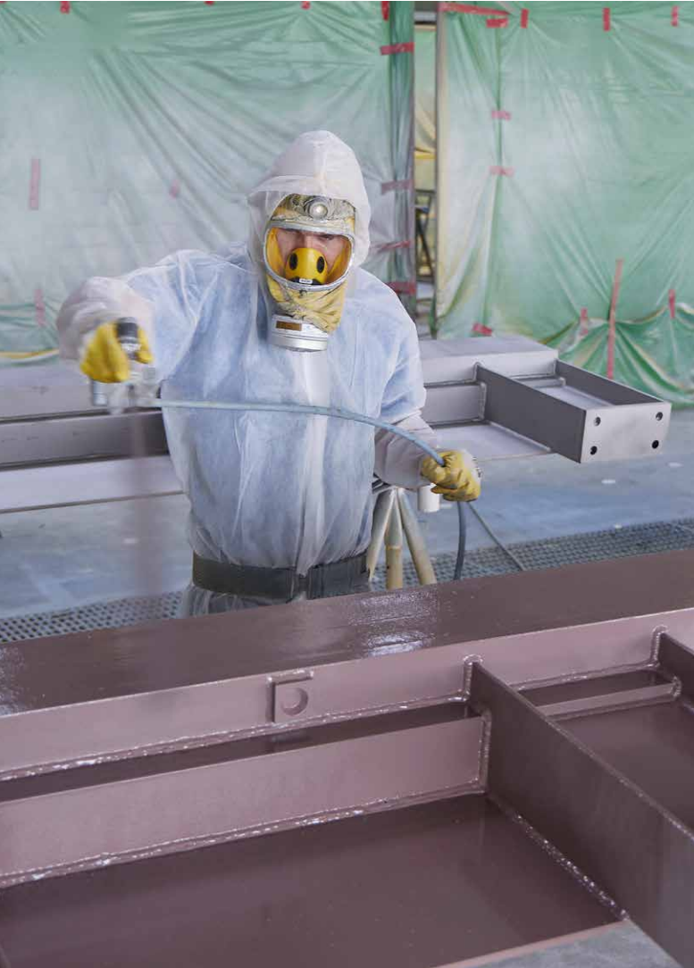
Application of surface protection on a steel structure
