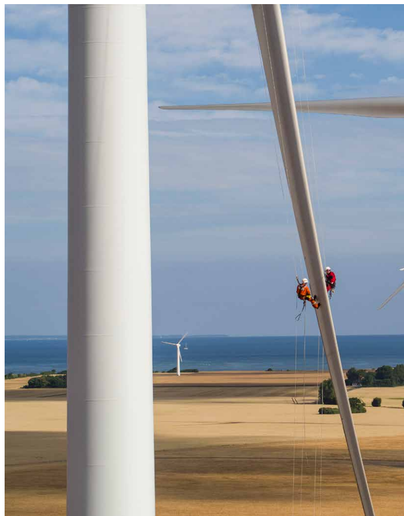
Inspection of coating on a wind turbine
