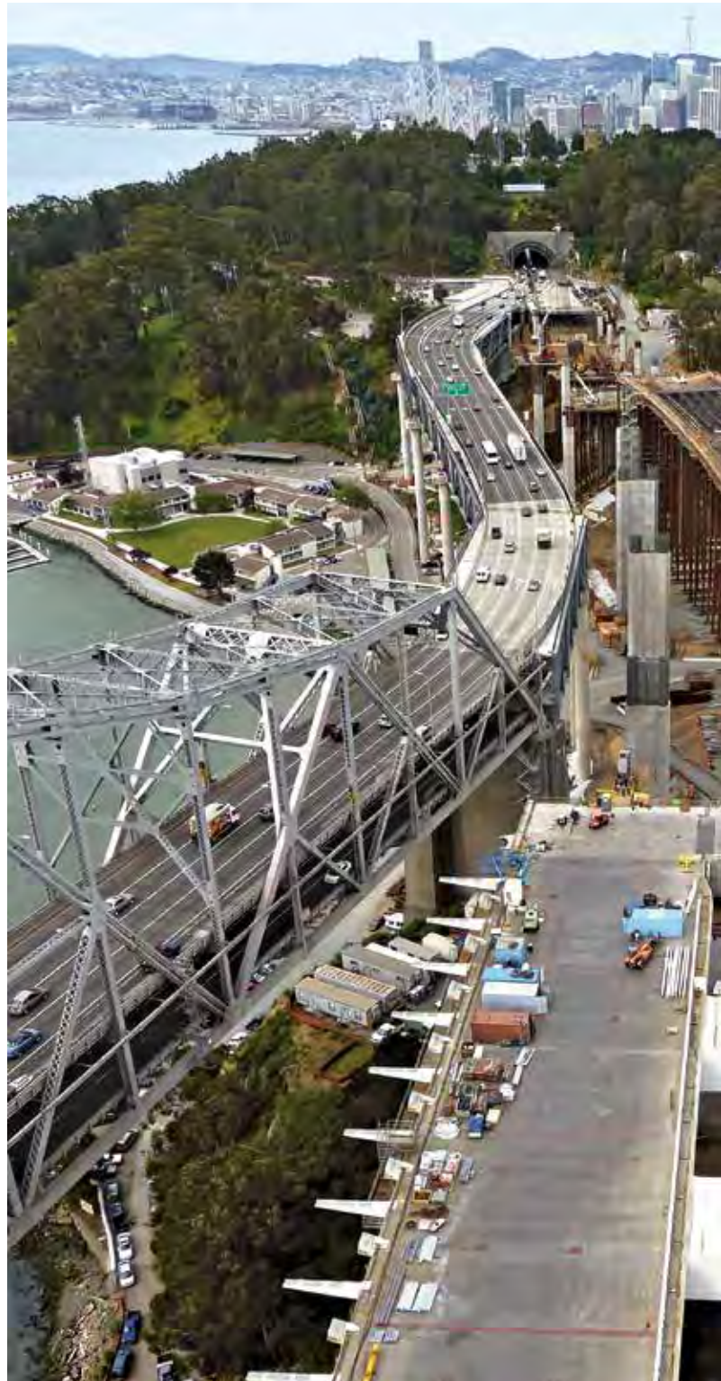
Oakland Bay Bridge, Kalifornien/USA
