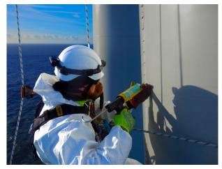
Servicing work on an offshore wind turbine
